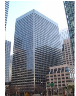
425 Market Street San Francisco, USA
